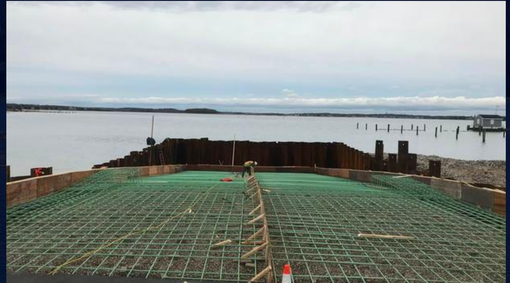
Cast In Place
