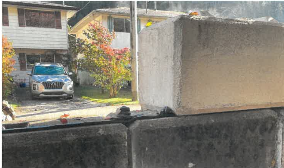
Figure 2: Mastic Sealant Applied to Floodwall
