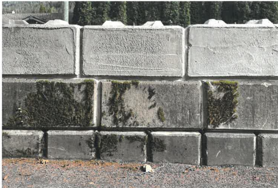
Figure 1: Flood Wall with Surface Sealant Applied
