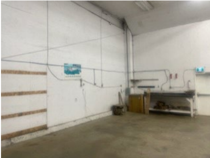
South east corner
