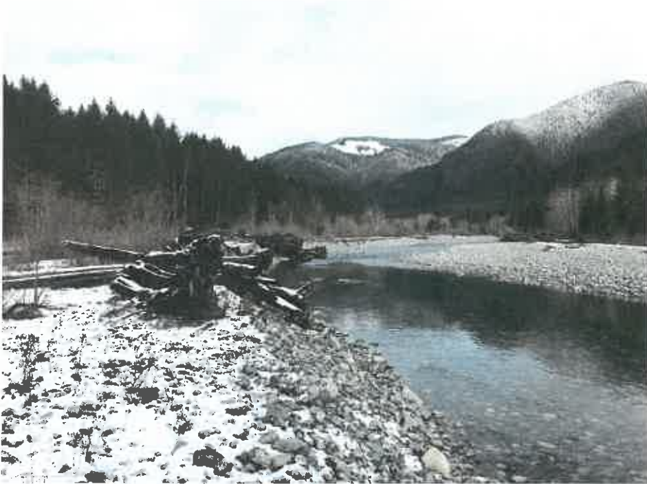
cabled root wads and LWD (2003) persist deflecting high flow toward thalweg
