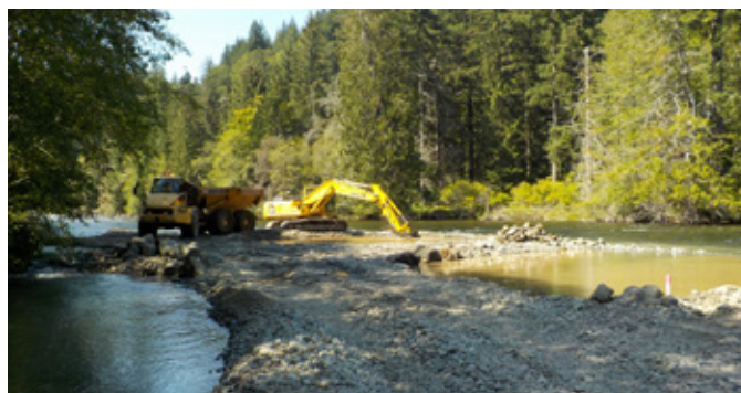
In the summer of 2019 with FWCP funding, 4,000 metric tonnes of gravel were placed 300 metres downstream of the John Hart Generating Station in the Campbell River area. The project, led by the Campbell River Salmon Foundation, has added 3,143 m 2 of Chinook salmon spawning habitat. It will also support coho, chum, and steelhead population. Photo courtesy of Campbell River Salmon Foundation.
