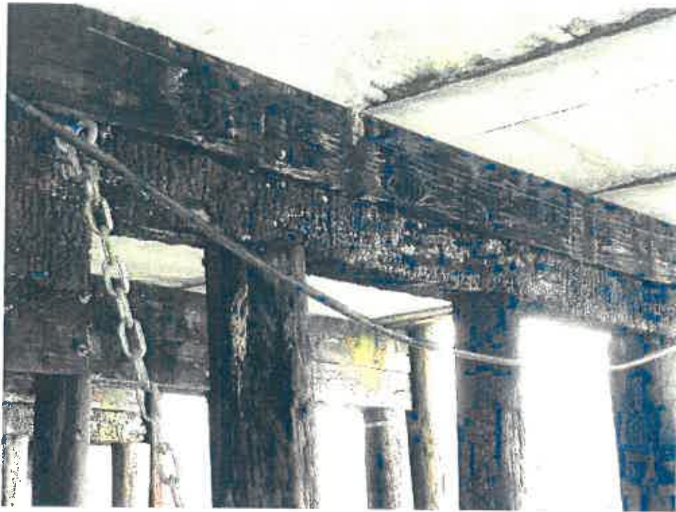
Photo 7 - Bent No. 7 Pile Nos. A to E: Lower Pile Cap with Severe Deterioration (South Face Shown). Lower pile cap has displaced north approximately 75mm to 100mm.
