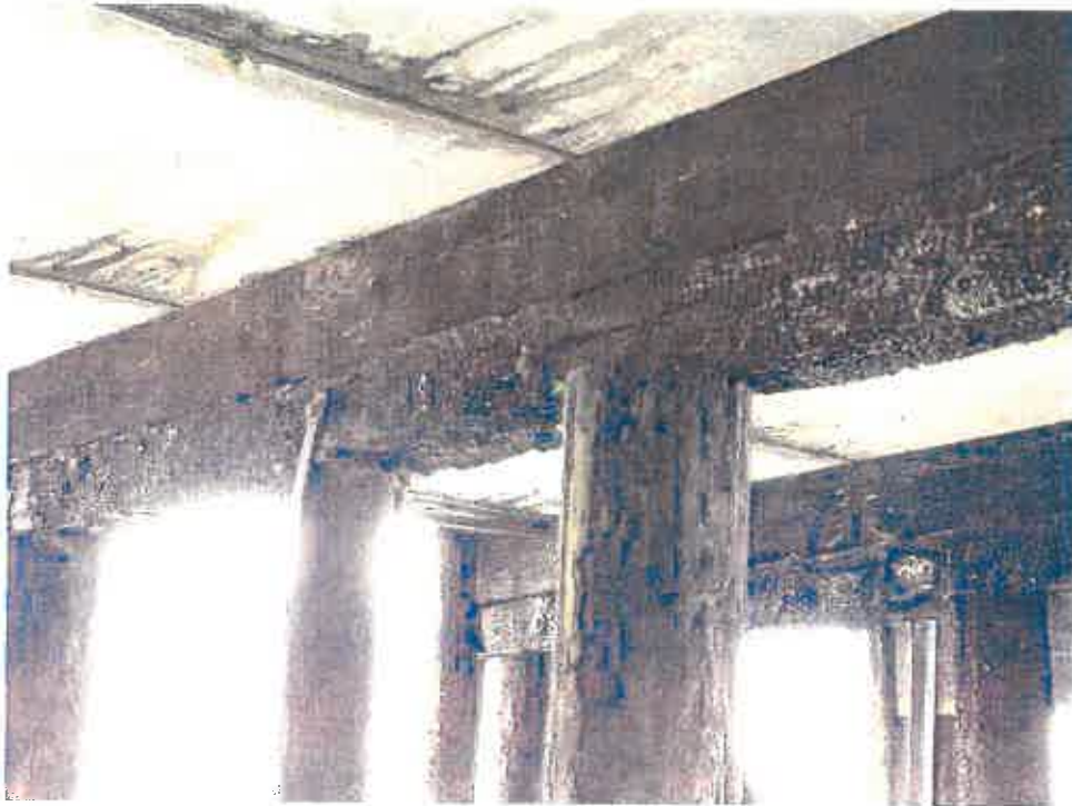
Photo 6 - Bent No. 6, Pile Nos. A to E: Lower Pile Cap with Severe Deterioration (North Face Shown). Lower pile cap has displaced north approximately 50mm.
