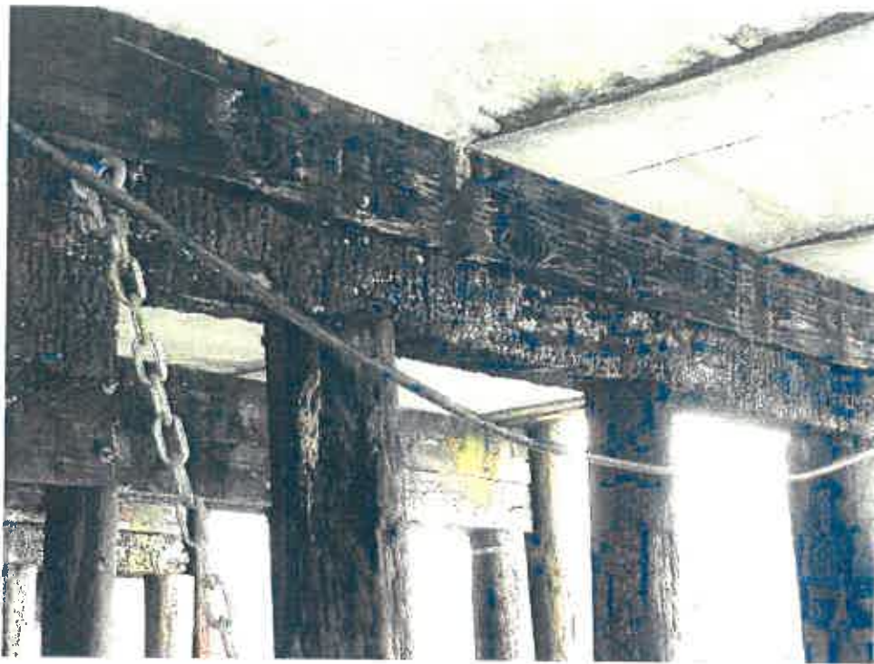
Photo 7 - Bent No. 7 Pile Nos. A to E: Lower Pile Cap with Severe Deterioration (South Face Shown). Lower pile cap has displaced north approximately 75mm to 100mm.
