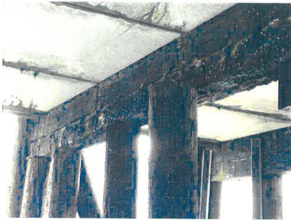
Photo 5 - Bent No. 5, Pile Nos. A to E: Lower Pile Cap With Severe Deterioration (North Face Shown). Lower pile is displaced north approximately 100mm.
