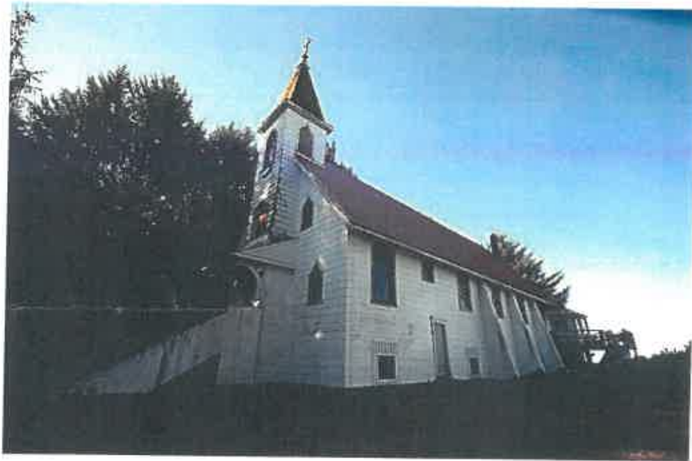
Yuquot Church, Summer 2016 (Photo: Macdonald & Lawrence)
