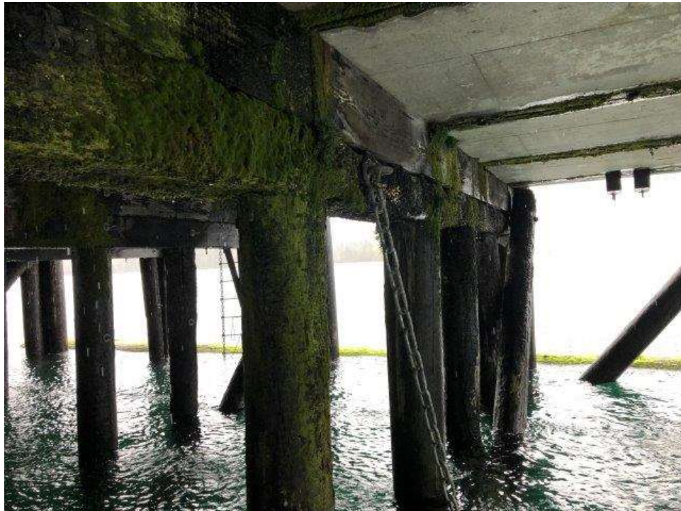
Photo 20 – Bent No. 2 Lower Pile Cap With Severe Fungal Decay
