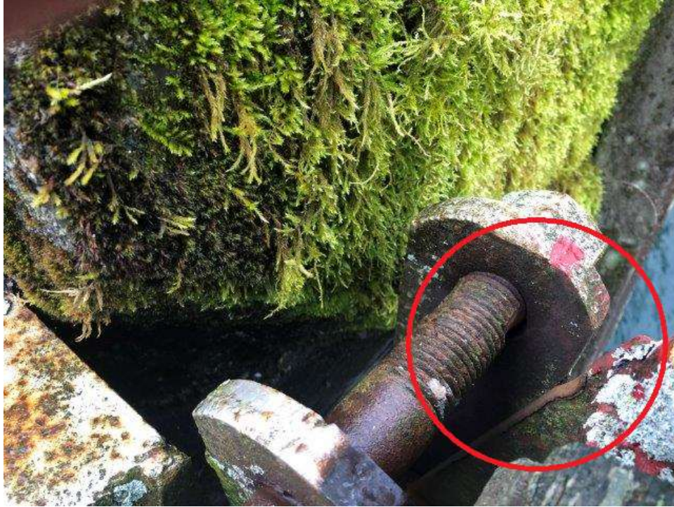
Photo 17 - West Hinge With Wearing / Abrasion of the Hinge Pin
