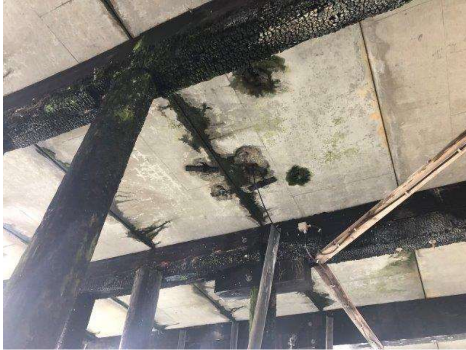
Photo 19 – Wharfhead Deck Panels With Spalling Adjacent to Drainage / Electrical Utility Holes
