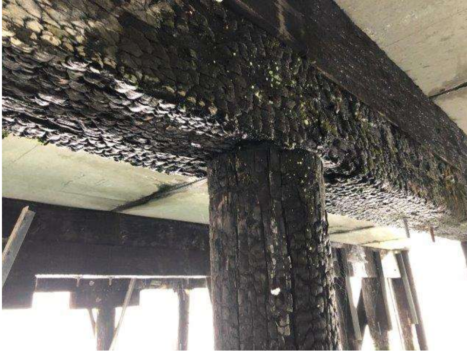
Photo 23 – Typical View of Pile “Punching” Through Pile Cap from Pile Cap Severe Fungal Decay
