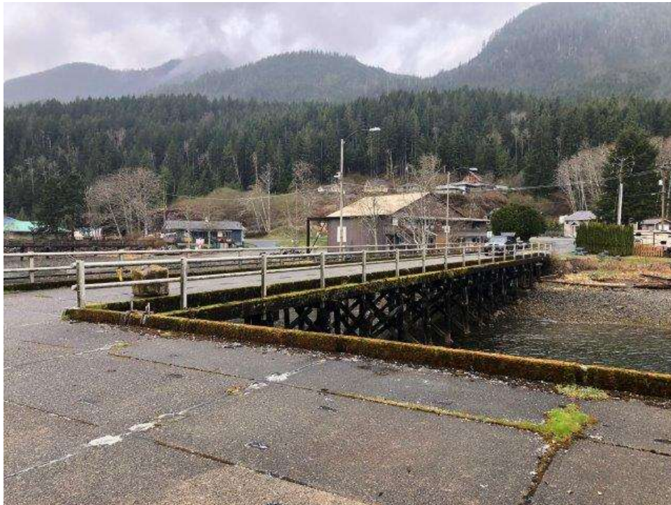
Photo 14 - No Handrails Along West Face of Wharfhead
