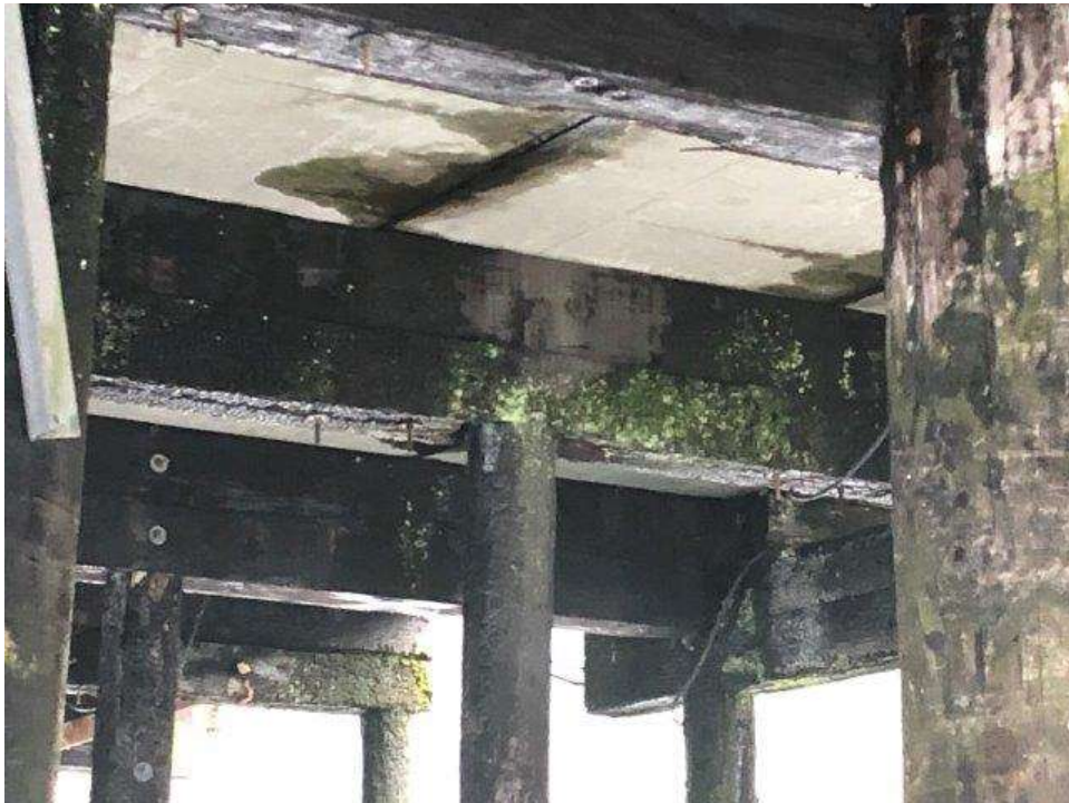
Photo 24 - Pile Punching Through Pile Cap at Pile No. 6T
