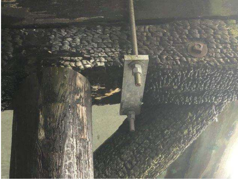
Photo 25 – Hiab Support Bracket to Pile Cap at Bent No. 13
