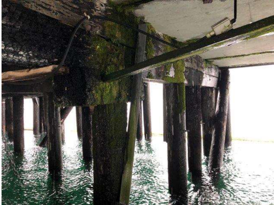
Photo 21 – Bent No. 3 Lower Pile Cap With Severe Fungal dEcay
