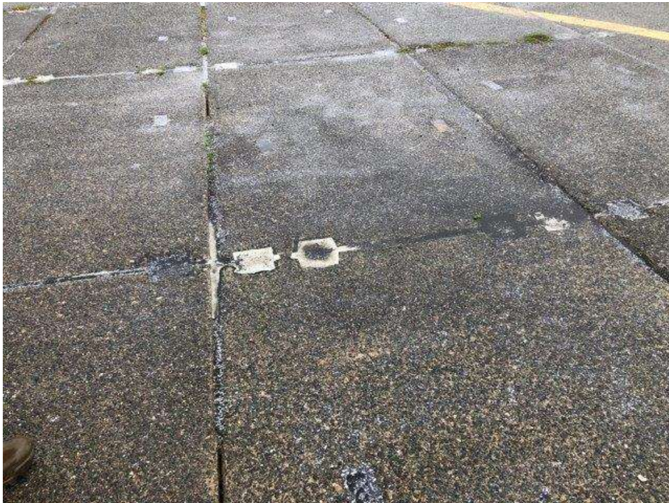
Photo 18 – Wharfhead Deck Panels with Settlement Due to Failure of the Pile Caps
